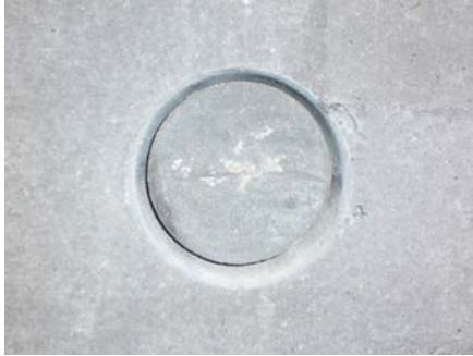
Color-matched plugs for anchor holes
