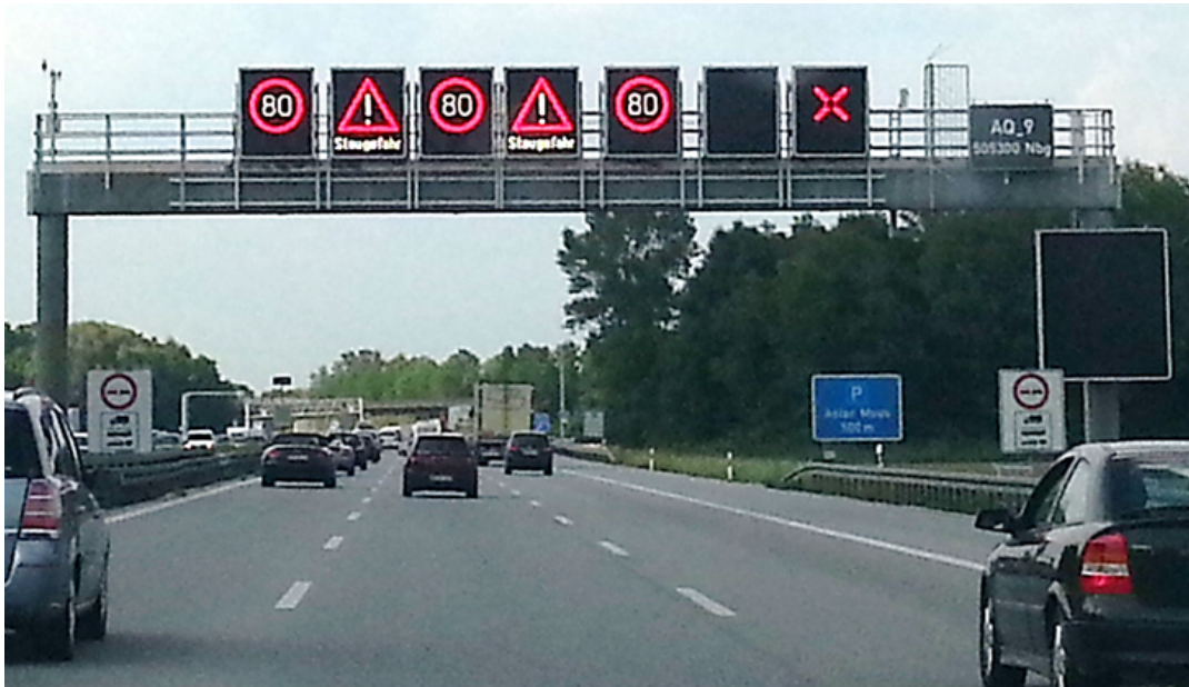
Figure 2.1: Example of VSL system in Germany.
