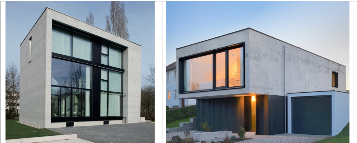
Figure 6 – Left: Private house Schlaich, Berlin, Germany. Right: Private house Thalmeier. Aiterbach, Germany
