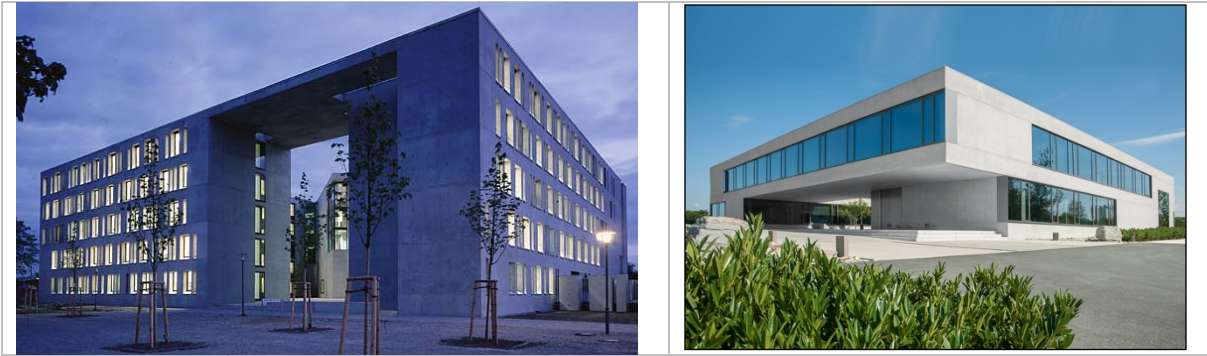
Figure 5 – Left: Regional and district court Frankfurt/Oder, Germany. Right: Office building, Erwitte, Germany
