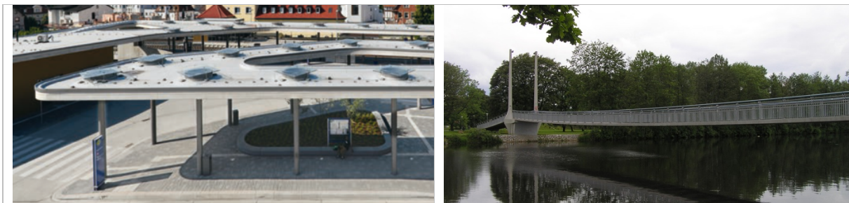
Figure 2 – Left: Bus station roof, Korbach, Germany. Right: Pedestrian bridge Budweis, Czech Republic
