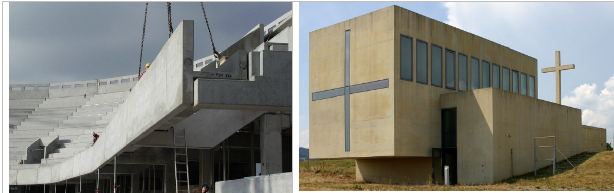
Figure 3 – Left: lower end element of the upper tribune, Volkswagen Arena, Wolfsburg, Germany. Right: Emmaus Autobahn chapel, rest and service area Hegau-West, Germany.
