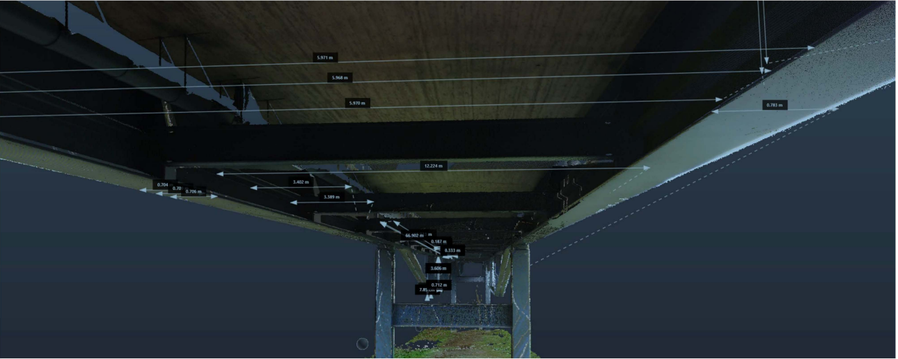
Figure 7: point cloud with extracted parameters of the cross section
