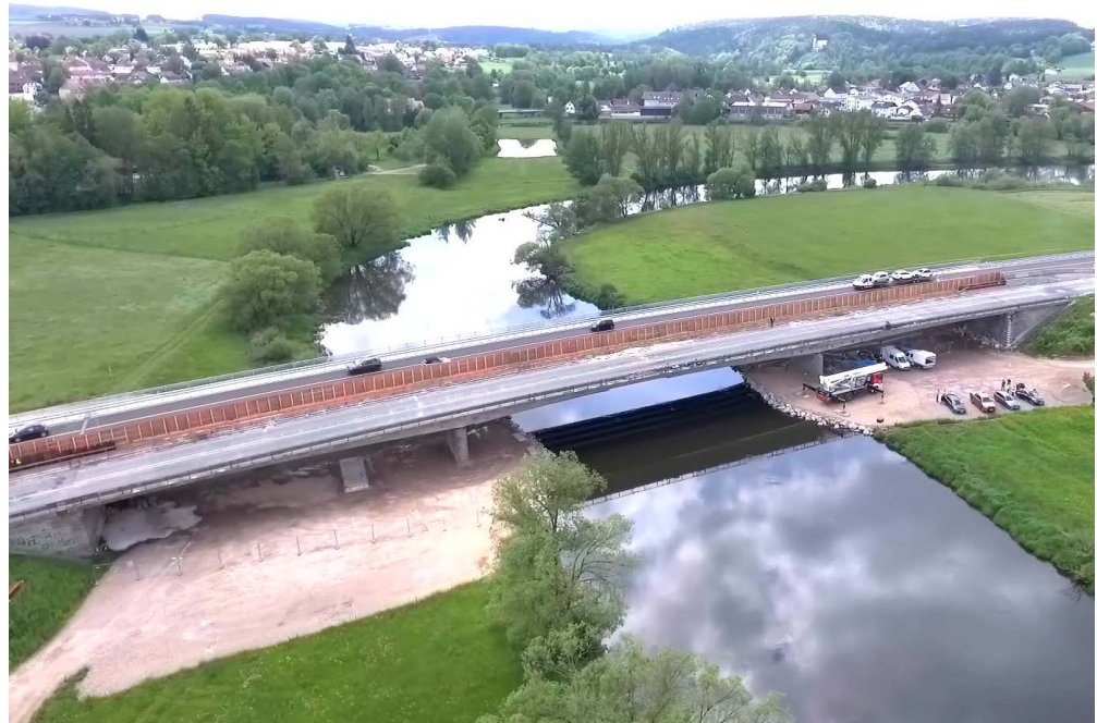
Figure 1. Overview screen of the test bridge in Roding from [21].
