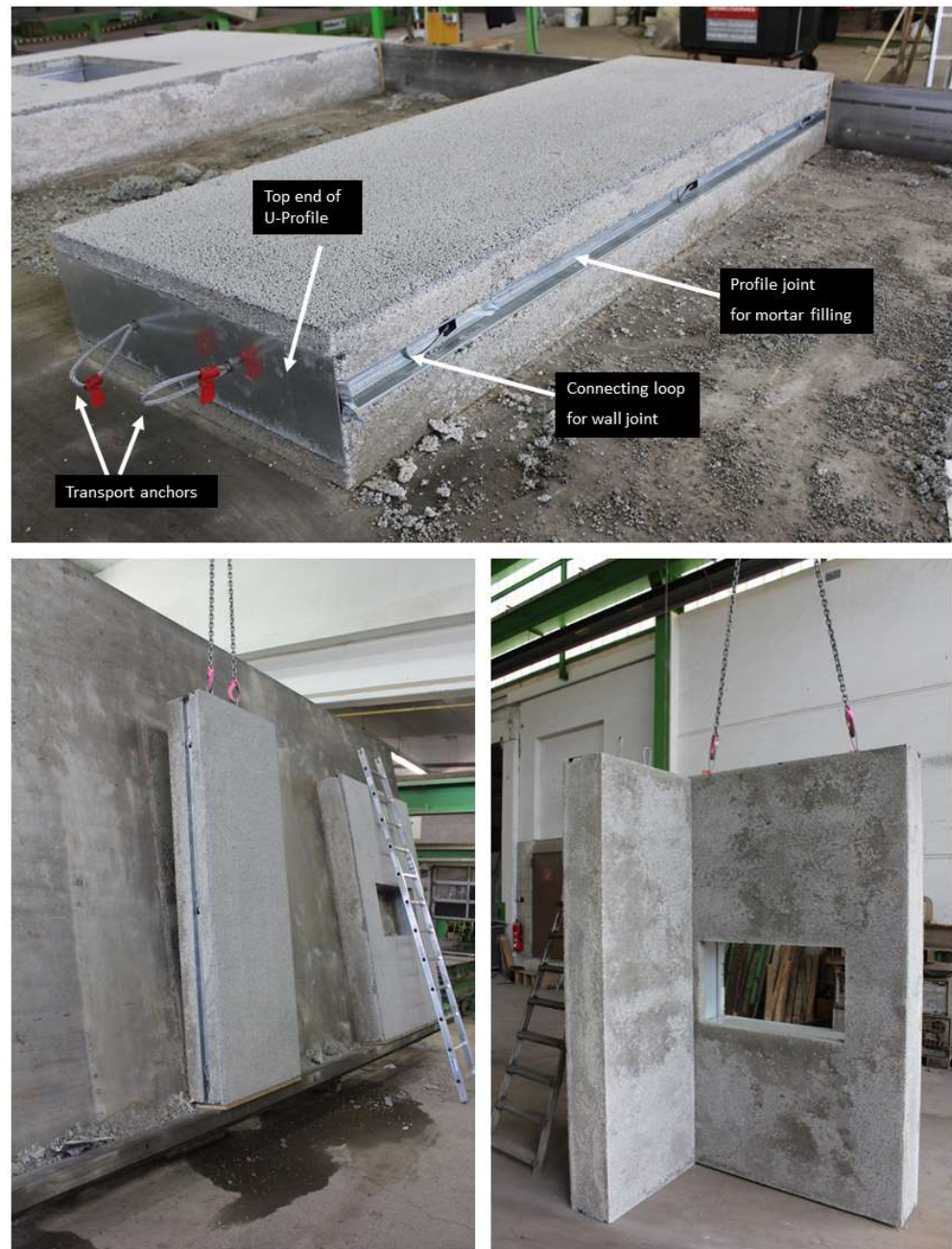
Figure 11. Connecting and anchoring elements for transporting, lifting, and connecting the individual precast elements.
