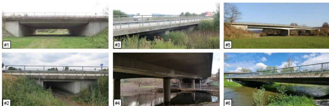
Figure 4: Investigated bridge structures within “ZfPStatik”-project, updated from [9]
