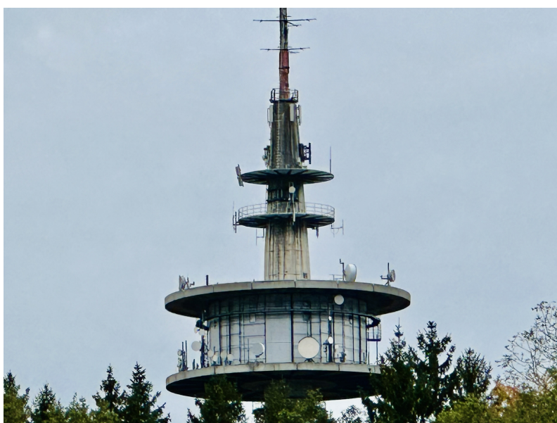
Figure 63: Photograph of the fixed service antennas on the radio tower in Schöngeising, Germany, located at 48.13199^{\circ} North, 11.22407^{\circ} East, from which fixed service interference was detected on 18th of October 2023 in the 18.2-18.7 GHz frequency band.
