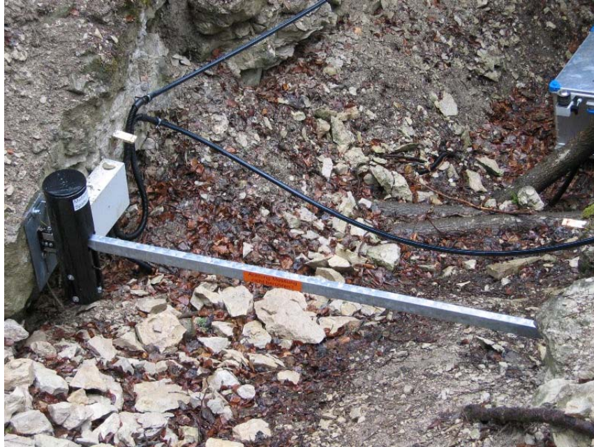
Figure 52: The on-site extensometer
