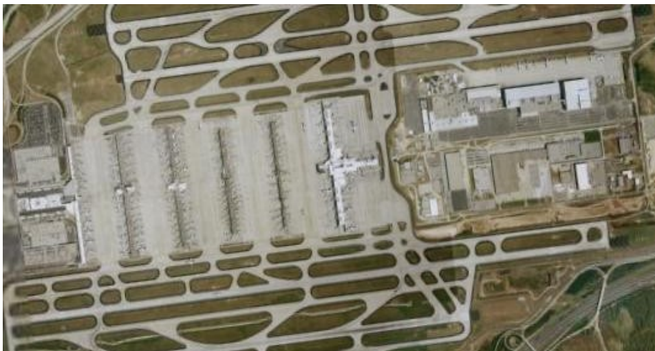
Atlanta International Airport - Luftbild (5-Ab-7)
