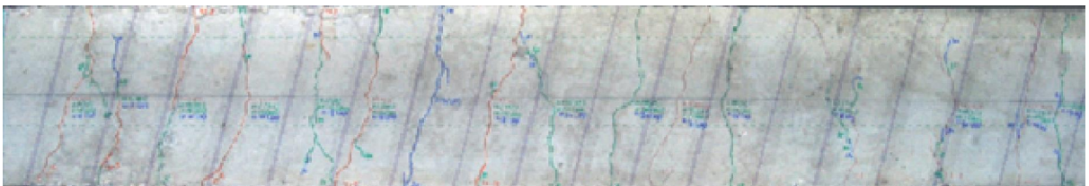
N3w2, loading 50kN, 64 % of Ultimate load
