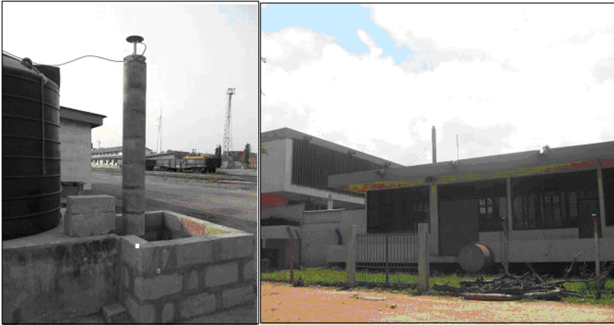
Figure 9-3 Pictures of the installed GNSS stations in Takoradi: TADI station (right); TKTG station (left)
